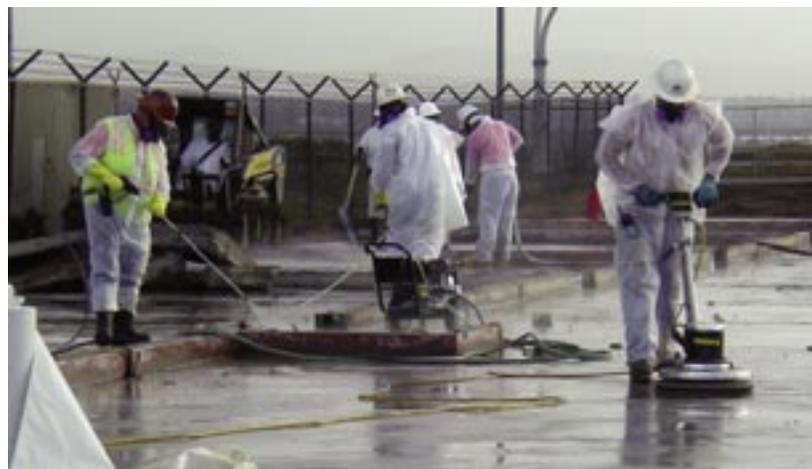
Workers polished concrete pads after tile removal.
